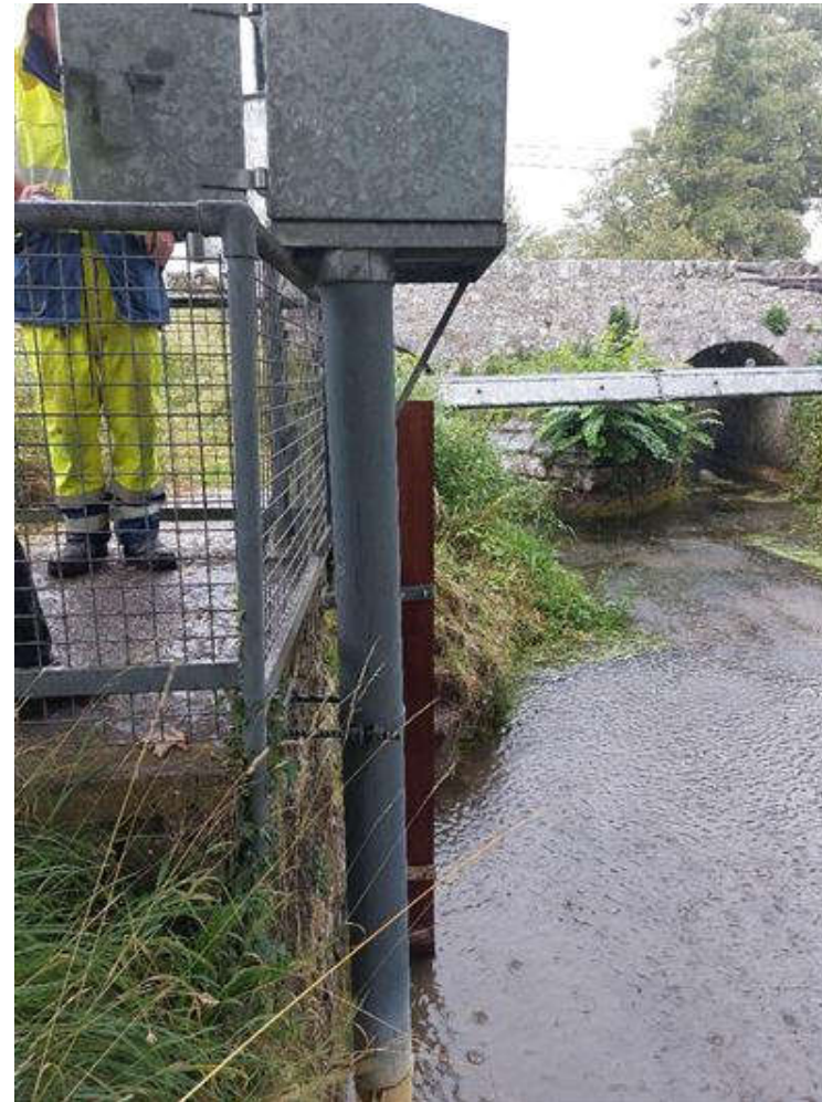
Plate 2 Aggard Bridge 29010 Hydrometric Station (facing downstream)
